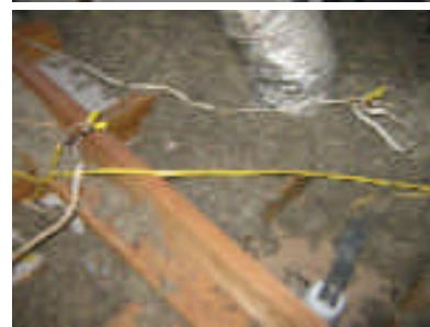
(a) There are spliced wires that need to be installed into a junction box at the rear right corner of the attic.
