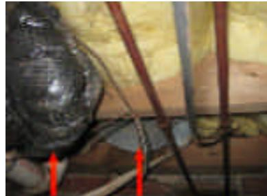
(h) There are heavy levels of moisture dripping off that air ducts in the crawl space. The temperature distribution may need to be adjusted or the ac unit is not functioning properly, have a licensed HVAC specialist evaluate and make repairs as needed.
