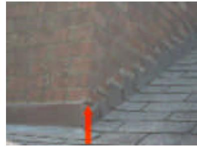
(g) The flashing needs to be sealed along the top of the garage roof where it meets the second story wall.
