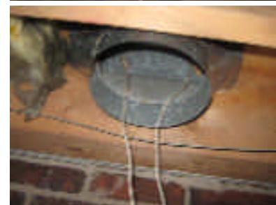
(d) There is standing water under the air ducts throughout the crawl space.
